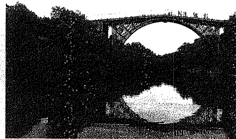
When England learned to make iron efficiently, the Industrial Age was born. It happened at Ironbridge Gorge. This is the first iron bridge ever built (1779).
